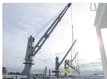
Synchronized Crane (50tons x 3)
